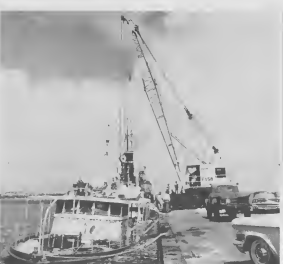
LAGO'S GIANT lift-ton crane had the Greyhound out of the water but had to lower her back to the harbor floor when her framing began breaking up under the strain. The hull of the wooden vessel was unreparable and tug eventually pulled the boat out to sea.
